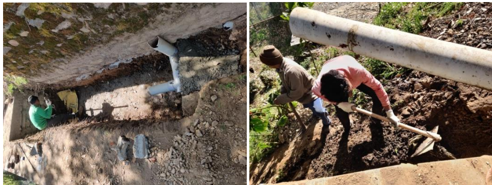
Grey water harvesting site- under the dining area to reuse water used for washing dishes
